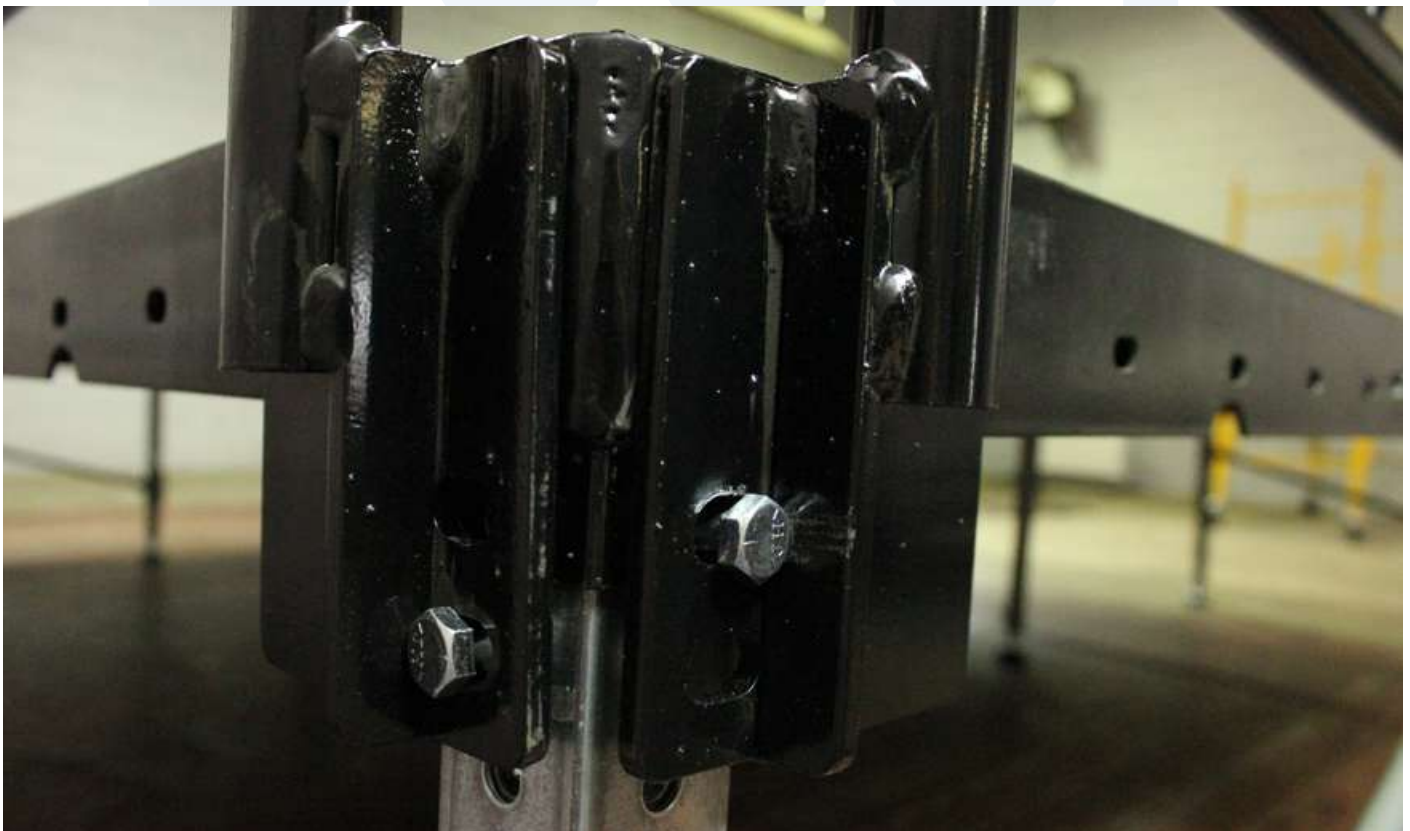
Closeup of guardrail attached to stage corner.
