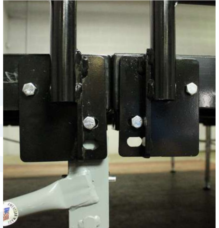
Closeup of guardrail attached to stage decks.
